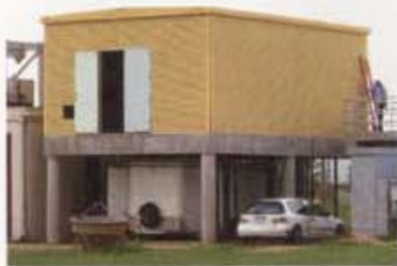
The elevated structure at Houston's Simms Bayou wastewater treatment plant protects key equipment such as pumps from potential floodwaters such as those which affected the city during Tropical Storm Allison in 2001.
